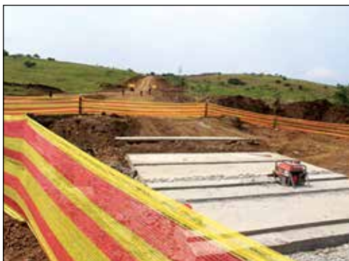
The soon to be completed Mlondo road in Ward 11, Cinci.
