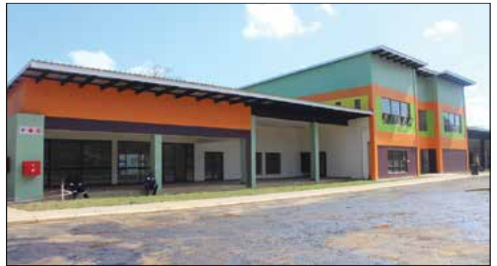
The newly finished Thusong Service Centre that will soon open to the public.
