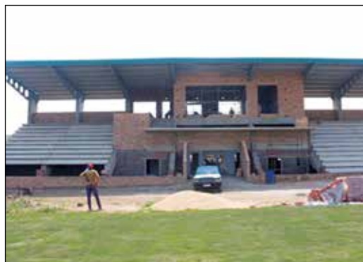
The soon to be completed stand for the Mawombe sport field.
